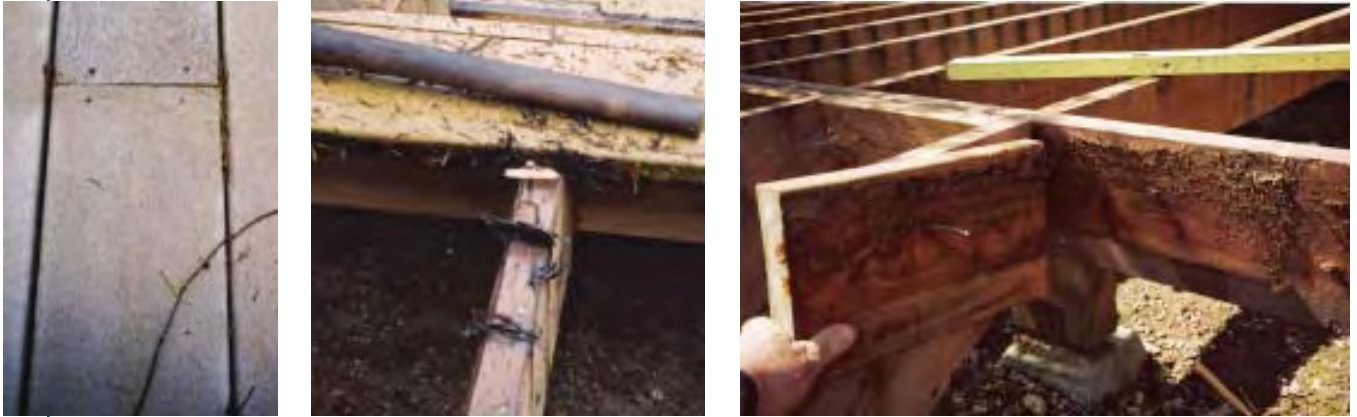
Figure 6. Most carpenters space deck boards too tightly (left), leaving enough room for debris to get in but no way to clean it out. On this deck, organic matter collected at every gap and joint (center), as well as between a rim joist and blocking that landed under a gap in the deck boards (right).
