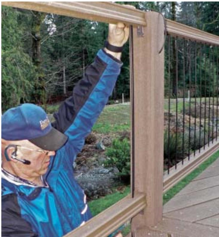
**Figure 3.** After installing the top rail, rods precut to the correct length help determine the bottom rail's height. With the rod bottomed out in the lower rail, the author raises the rail until he feels the rod become flush with the top of the upper rail. That's when he screws home the lower rail's support bracket.
