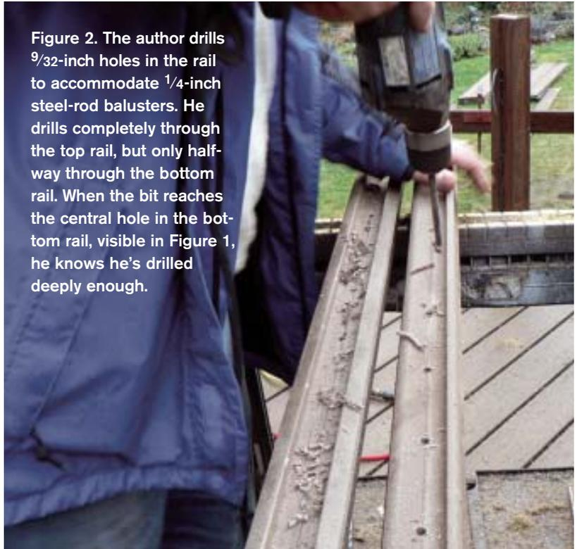
**Figure 2.** The author drills  $\frac{9}{32}$ -inch holes in the rail to accommodate  $\frac{1}{4}$ -inch steel-rod balusters. He drills completely through the top rail, but only halfway through the bottom rail. When the bit reaches the central hole in the bottom rail, visible in Figure 1, he knows he's drilled deeply enough.
